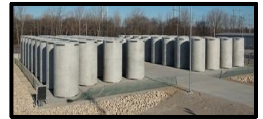
Temp. Storage Casks
